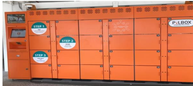
SHP-Tampines (L1 - near the side gate) 1, Tampines Street 41, S(529203)
